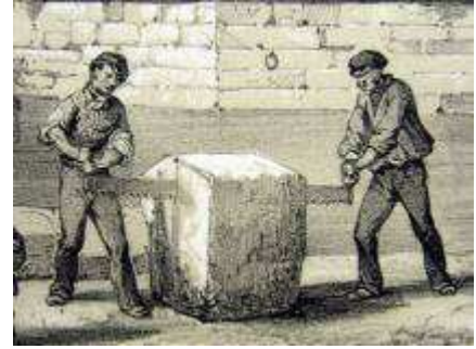
Stone cutters, detail of the engraving Apse of St Pierre's Church in Caen.-1852 (Musée de Normandie)
